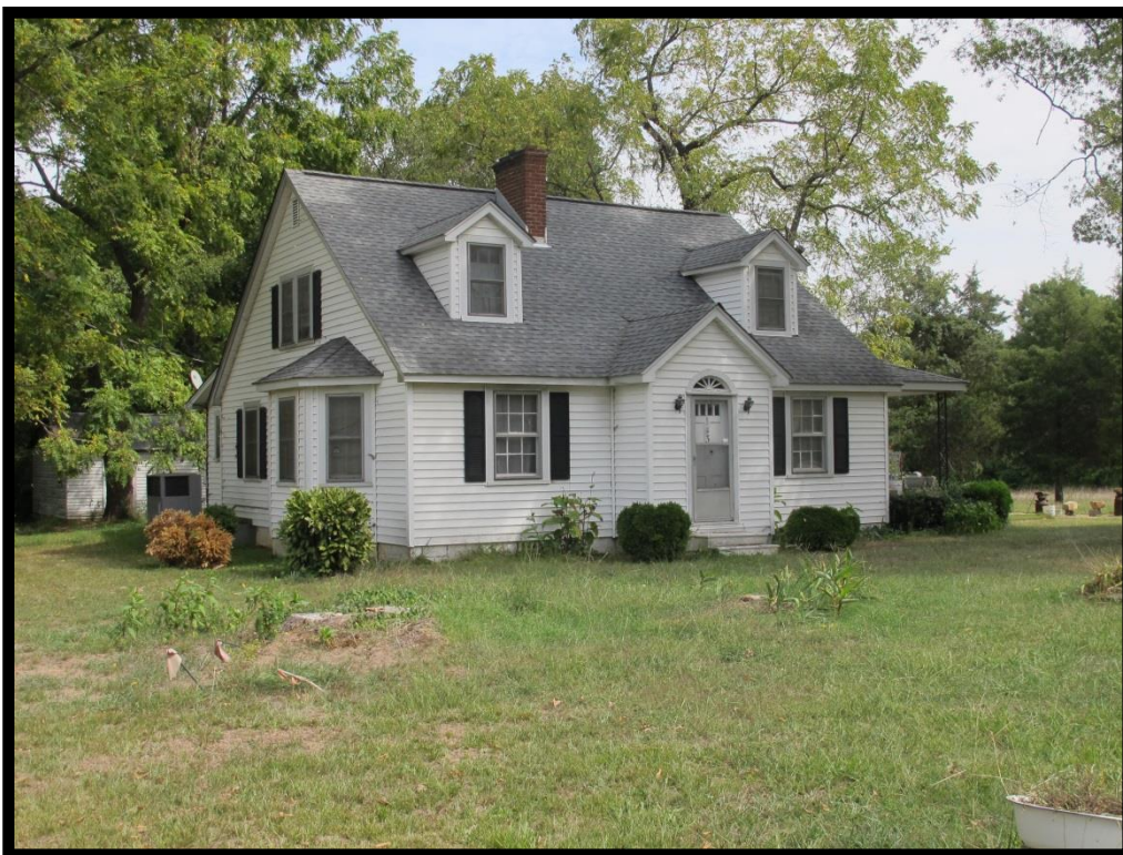
162 – View of House, 143 S. Church Street Looking Southeast
