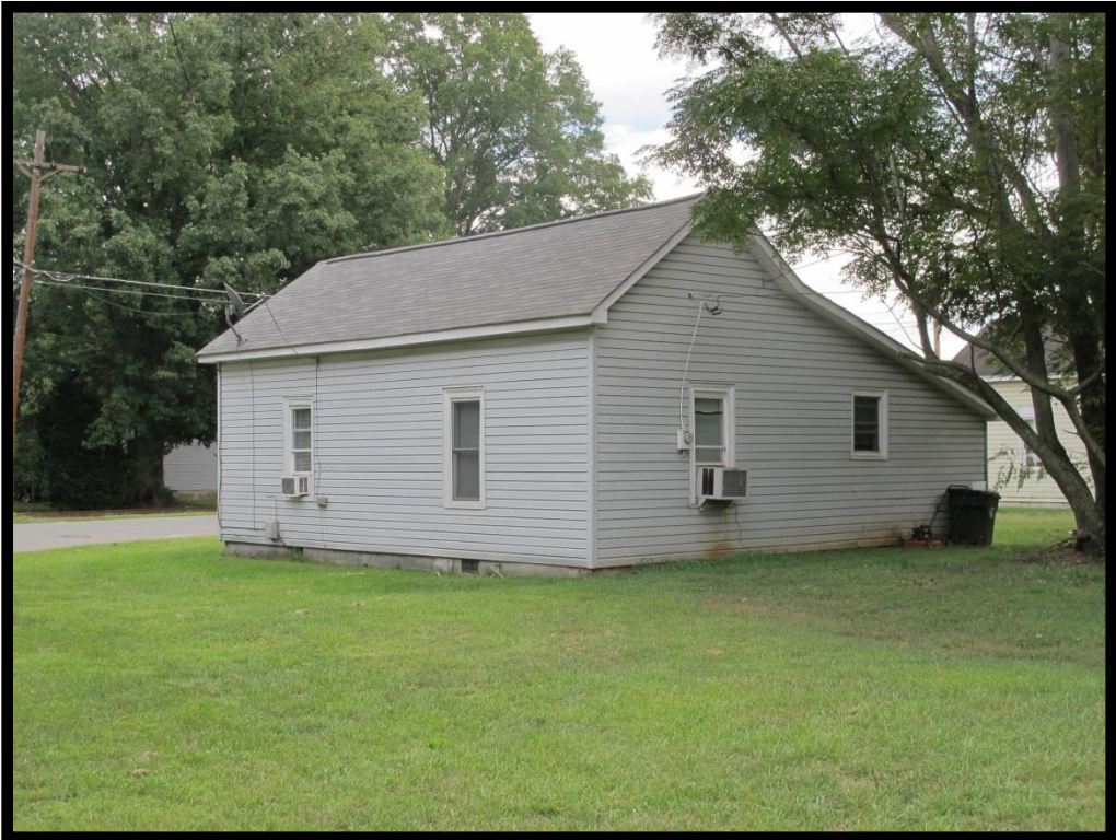
005 – View of House, 311 N Main St Looking Southeast
