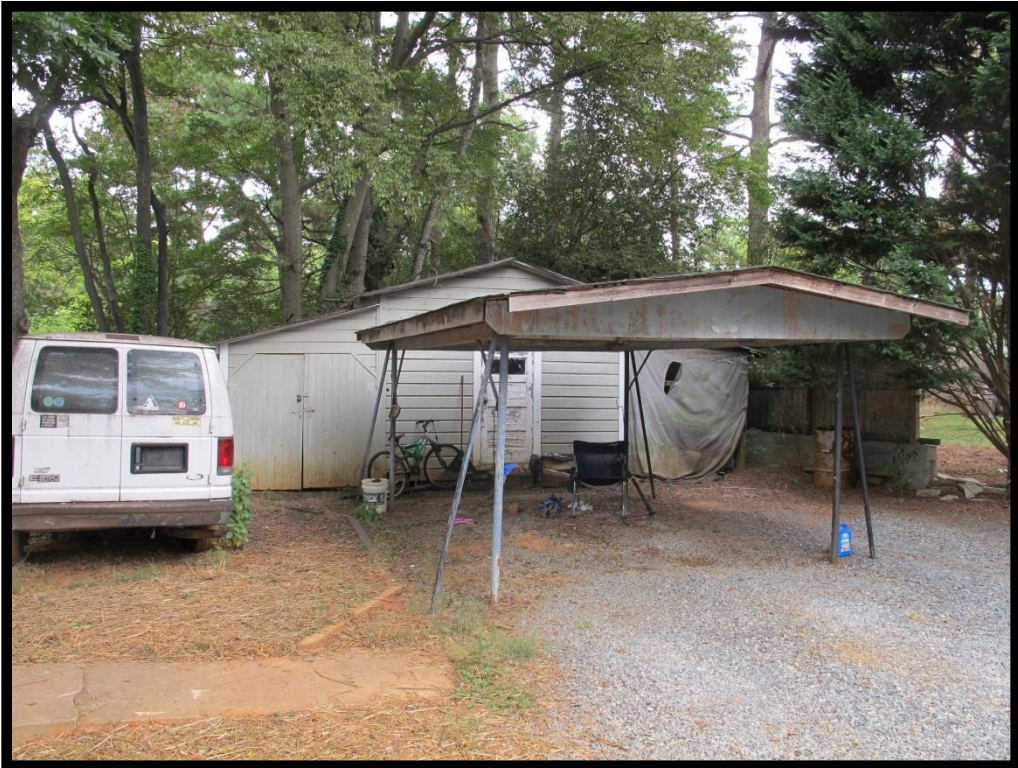
009 – View of Ancillary Structure at House, 105 W Church St Looking Northeast
