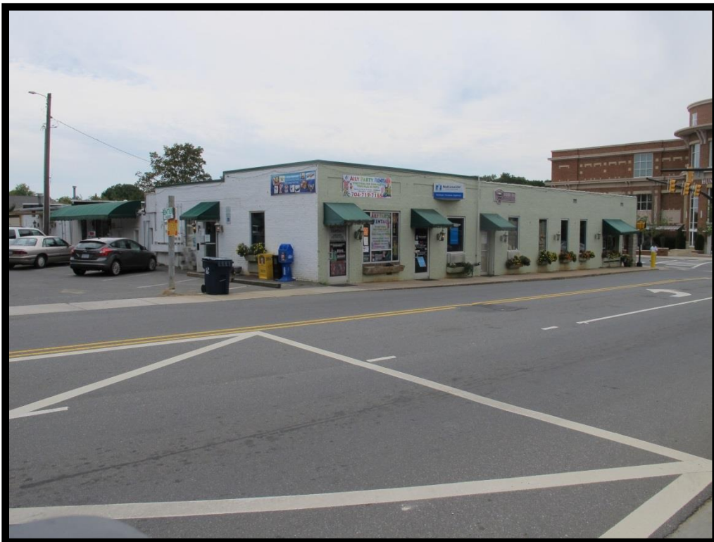
023 – View of Commercial Building, 101 S Old Statesville Rd Looking Southwest
