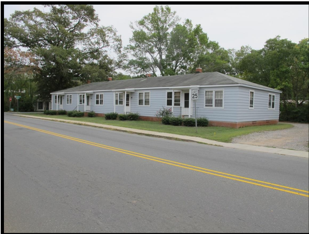
222 – View of Apartment Building, 104 Huntersville-Concord Road Looking Southwest
