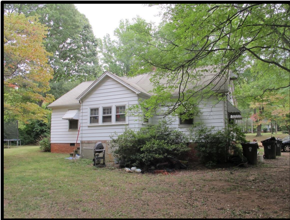
004 – View of McGinnes House, 401 N Old Statesville Rd Looking Northeast
