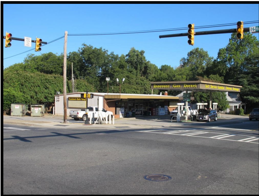
022 – View of Convenience Store/Gas Station, 101 N Old Statesville Rd Looking Northwest
