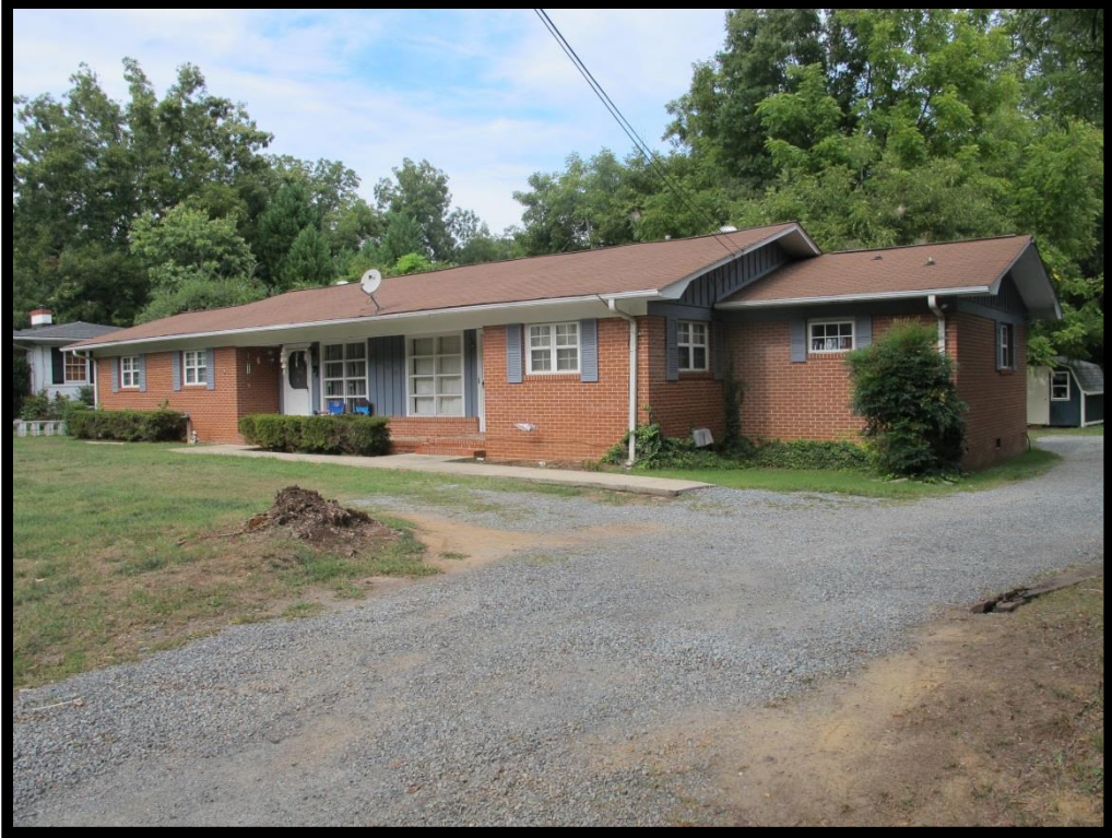
034 – View of House, 505 S Old Statesville Rd Looking North
