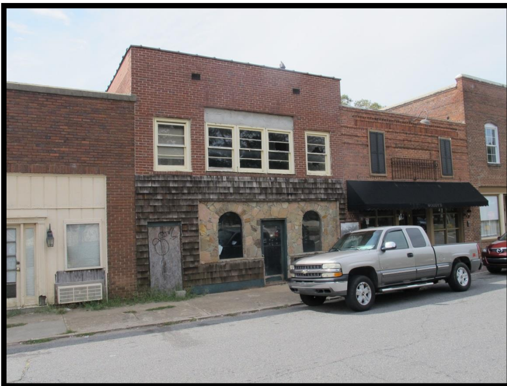
157 – View of Commercial Buildings 110 S. Main Street Looking Northwest
