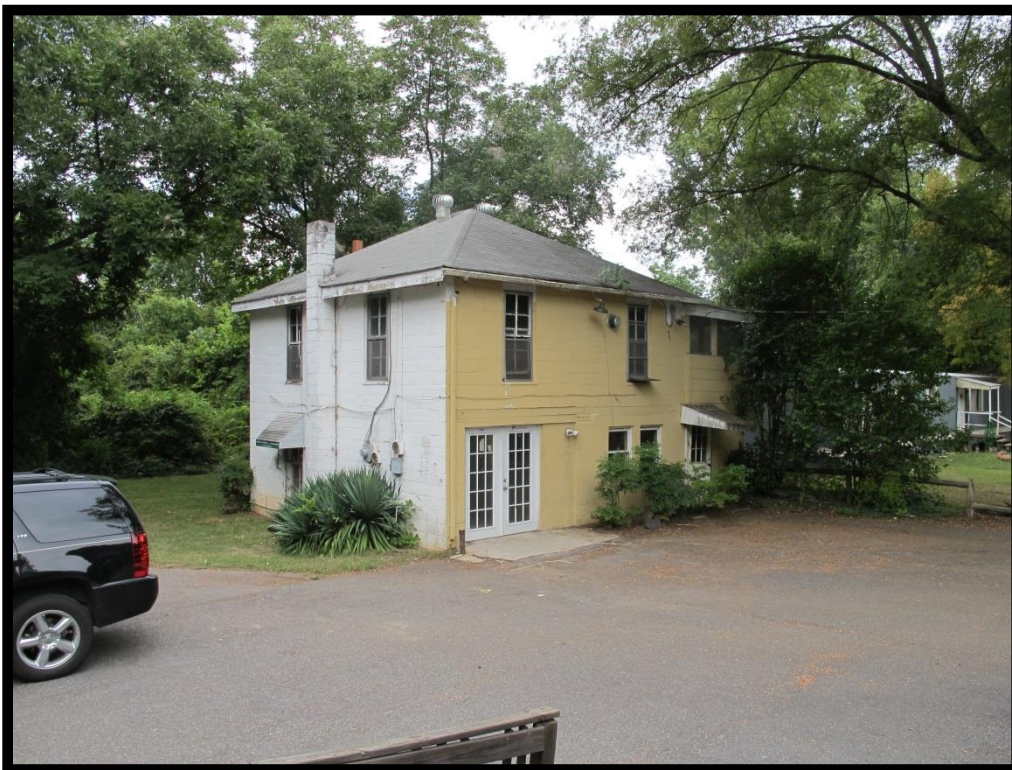
003 – View of Ancillary Structure at (former) House, 403 N Old Statesville Rd Looking Northwest
