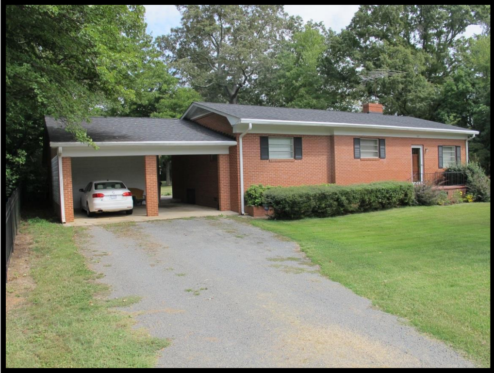
030 – View of House, 207 S Church St Looking Southeast
