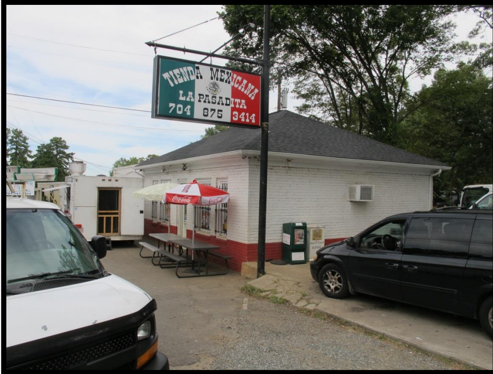
002 – View of Commercial Buildings, 500 N Old Statesville Rd Looking Northeast
