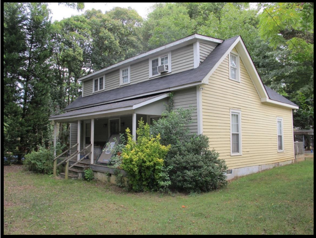
009 – View of House, 105 W Church St Looking Northeast
