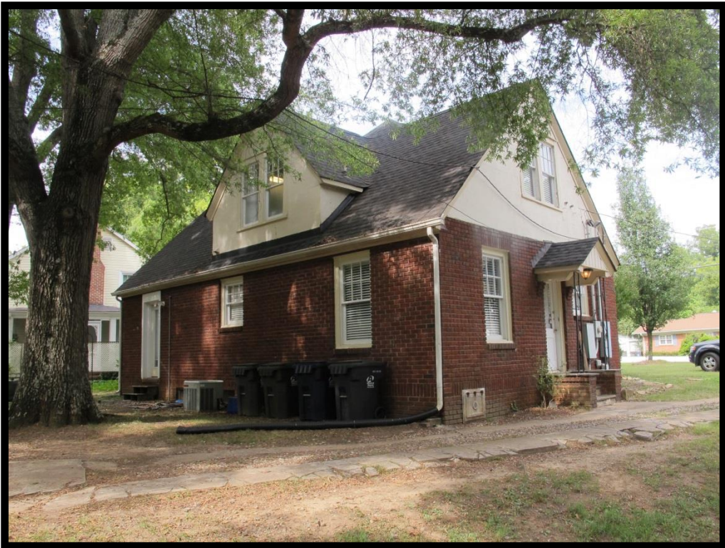
033 – View of House, 506 S Old Statesville Rd Looking Northwest
