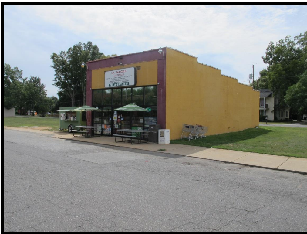
158 – View of Commercial Building, 116 S. Main Street Looking Southwest
