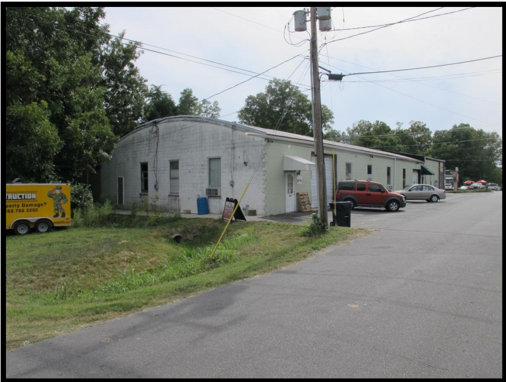
038 – View of Commercial Building, 501 S Old Statesville Rd Looking Southwest
