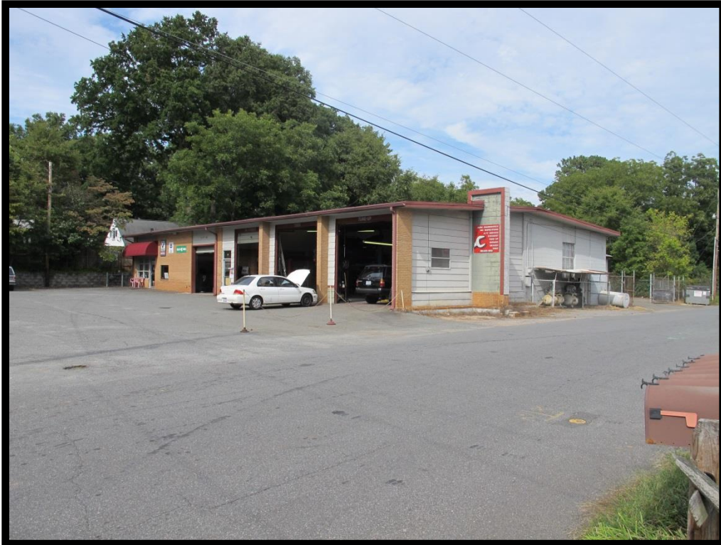
042 – View of Garage, 411 S Old Statesville Rd Looking Northeast
