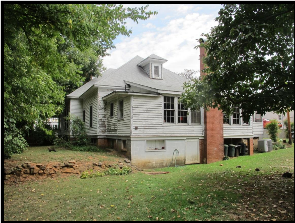
021 – View of House, 103 N Old Statesville Rd Looking Southeast
