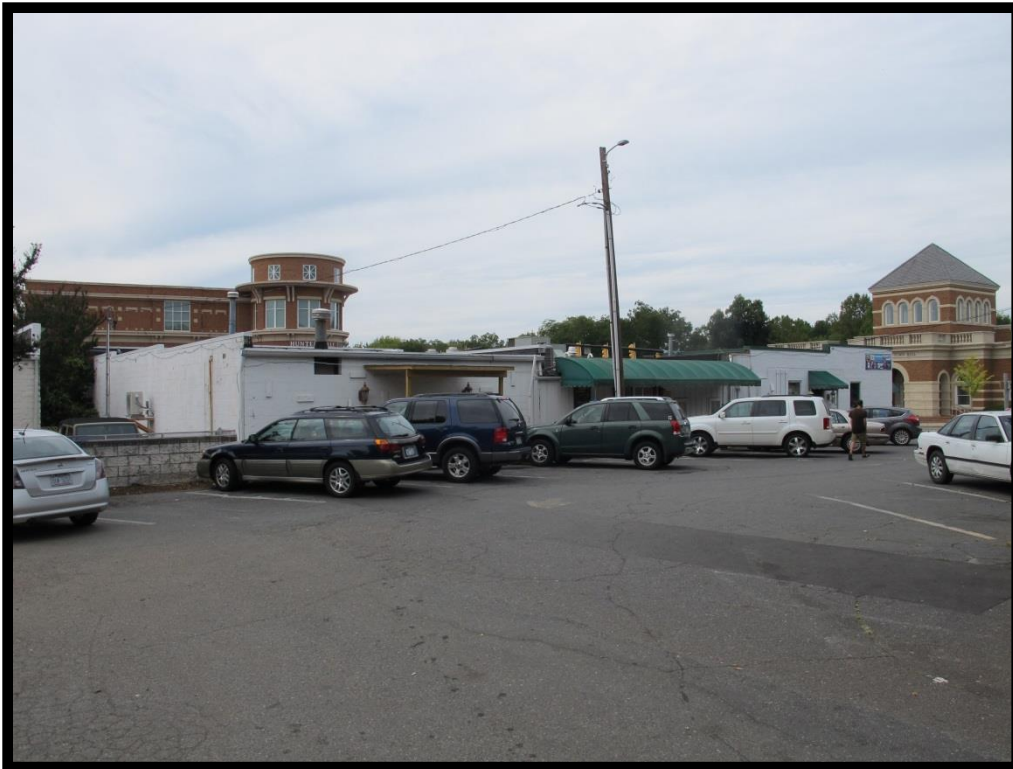
025 – View of Commercial Building, 105 S Old Statesville Rd Looking Northwest
