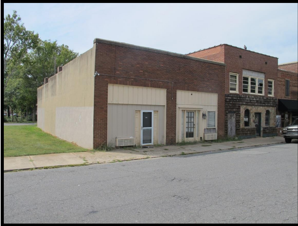
157 – View of Commercial Building 114 S. Main Street Looking Northwest
