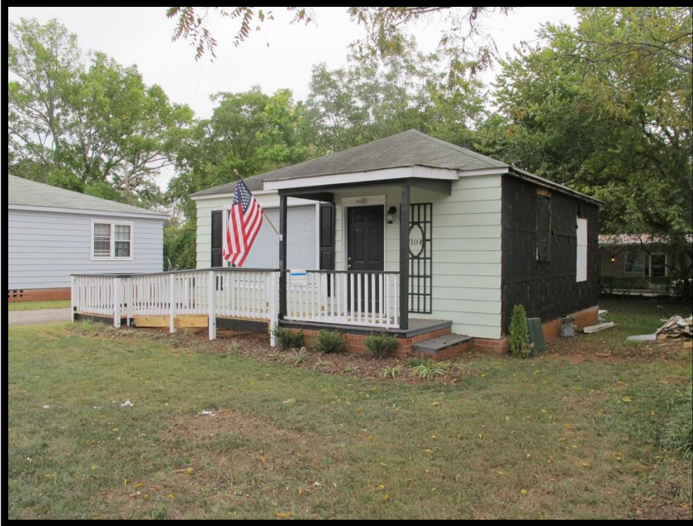
222 – View of Apartment Building, 104 Huntersville-Concord Road Looking Southwest
