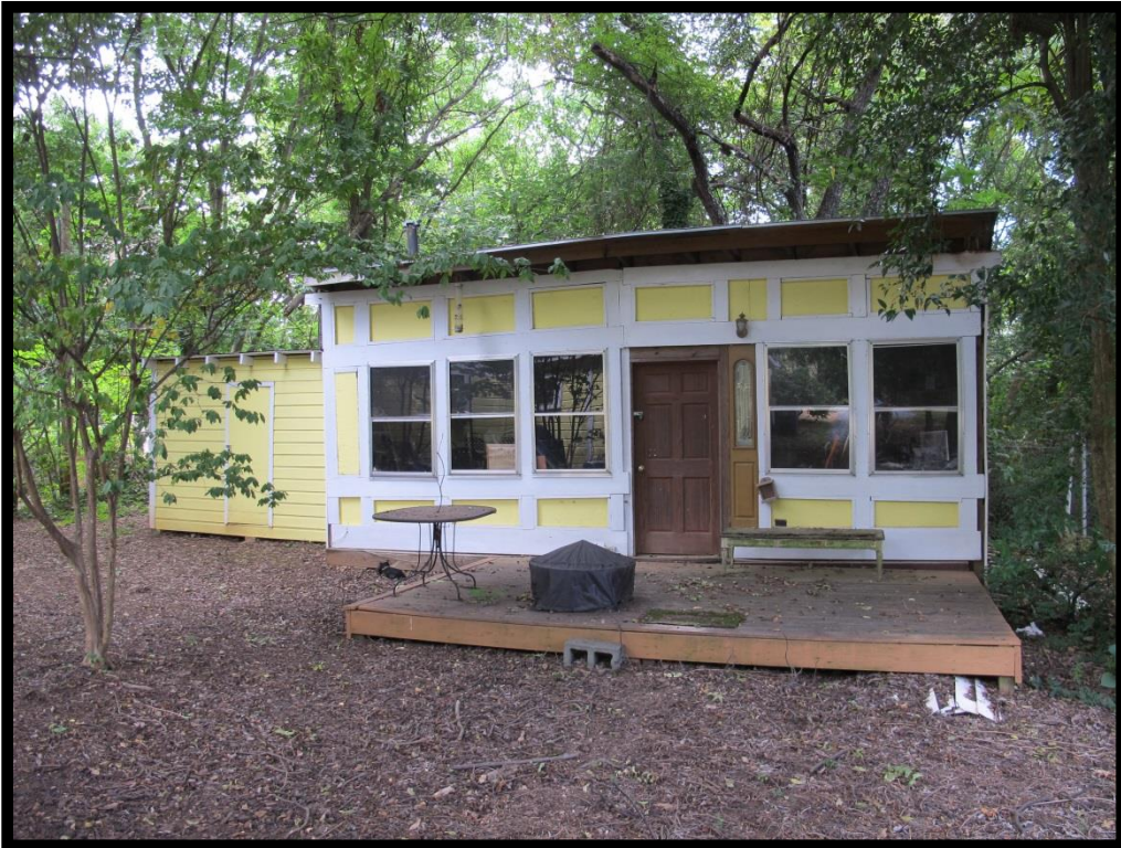
012 – View of Ancillary Structures at House, 102 W Church St Looking Southeast
