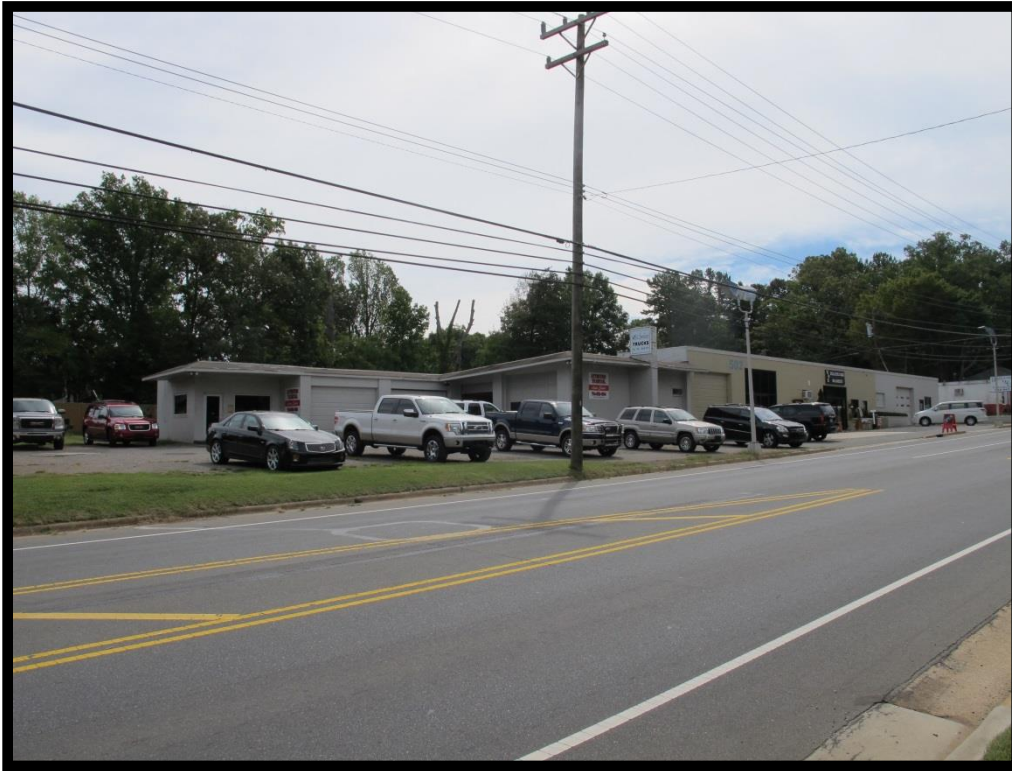
001 – View of (former) AMC Dealership, 502 N Old Statesville Rd Looking Southeast
