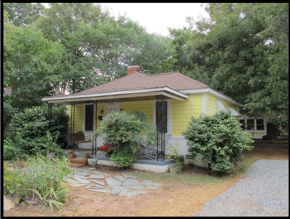
012 – View of House, 102 W Church St Looking Southeast
