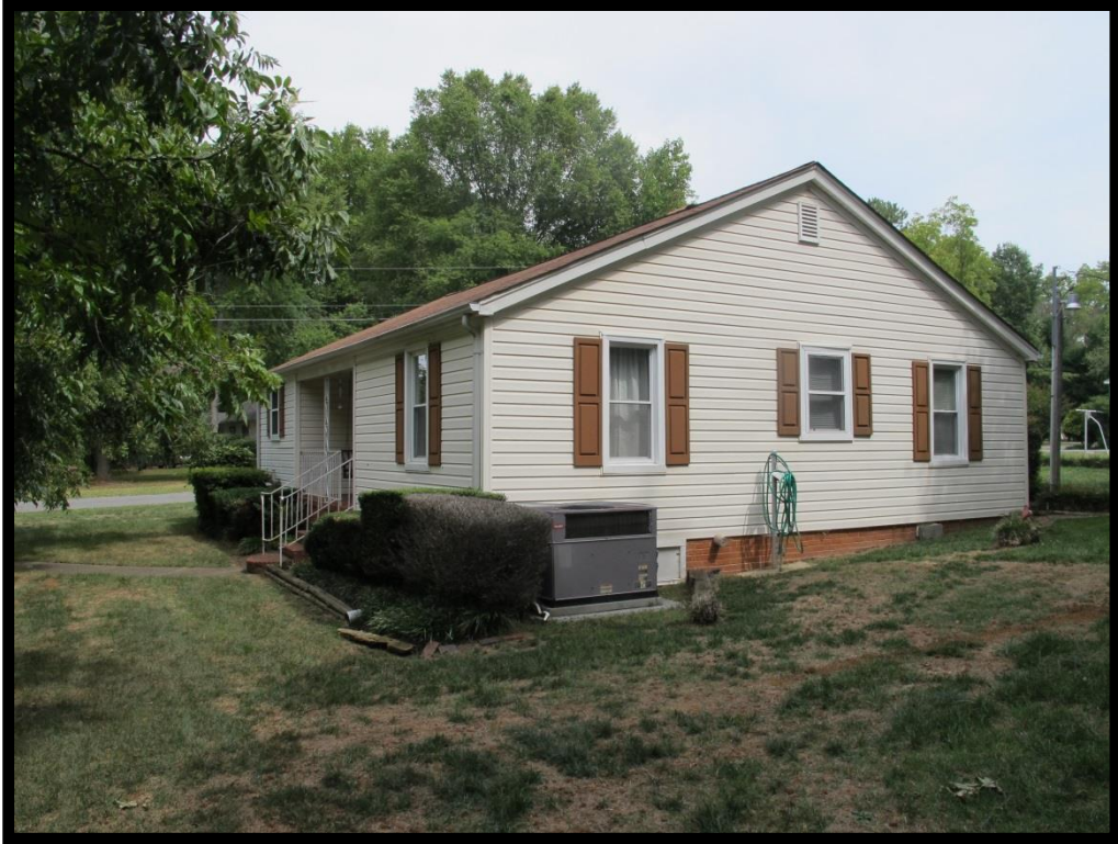
010 – View of House, 306 N Old Statesville Rd Looking Northeast
