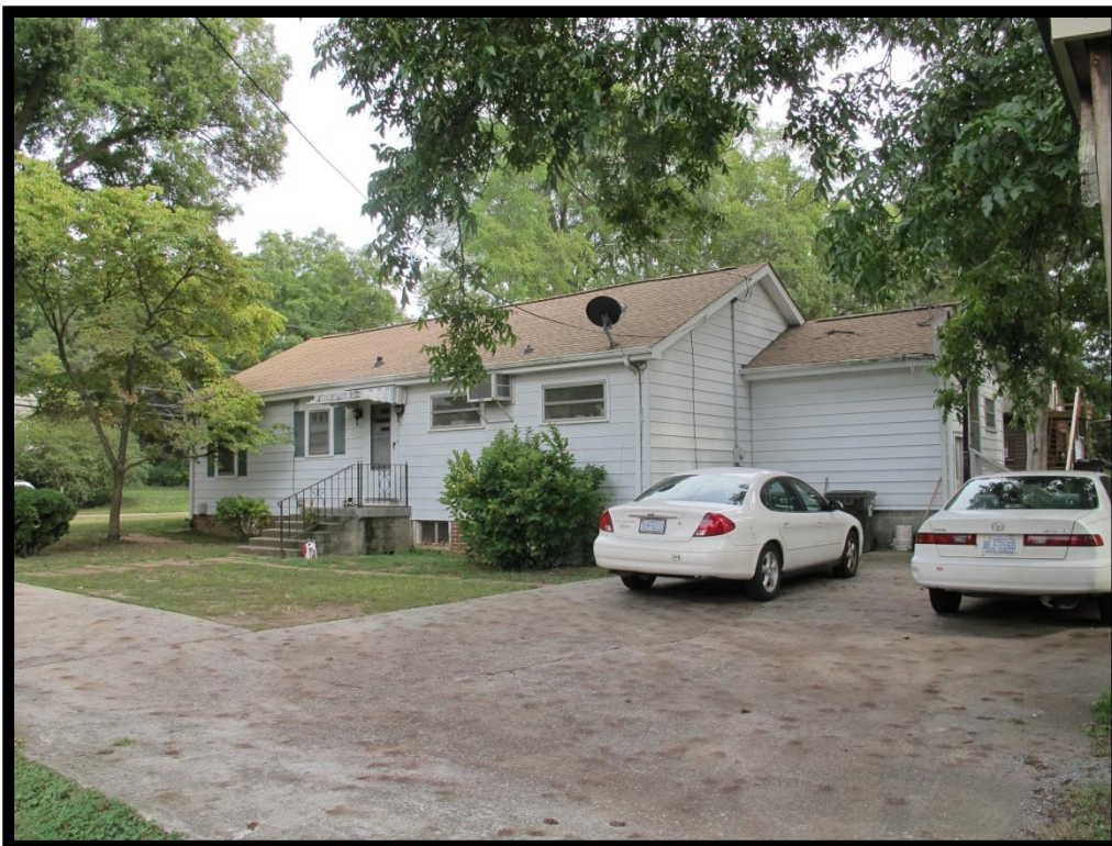
048 – View of House, 406 S Old Statesville Rd Looking Southeast
