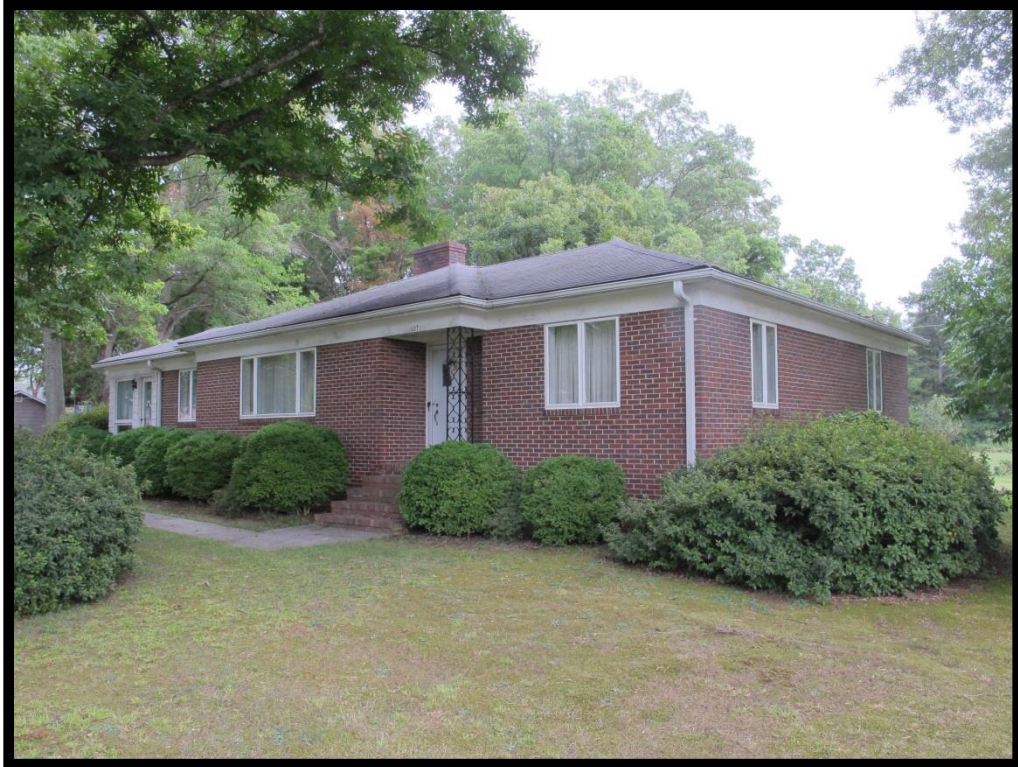
041 – View of House, 107 Mt Holly-Huntersville Rd Looking Southeast
