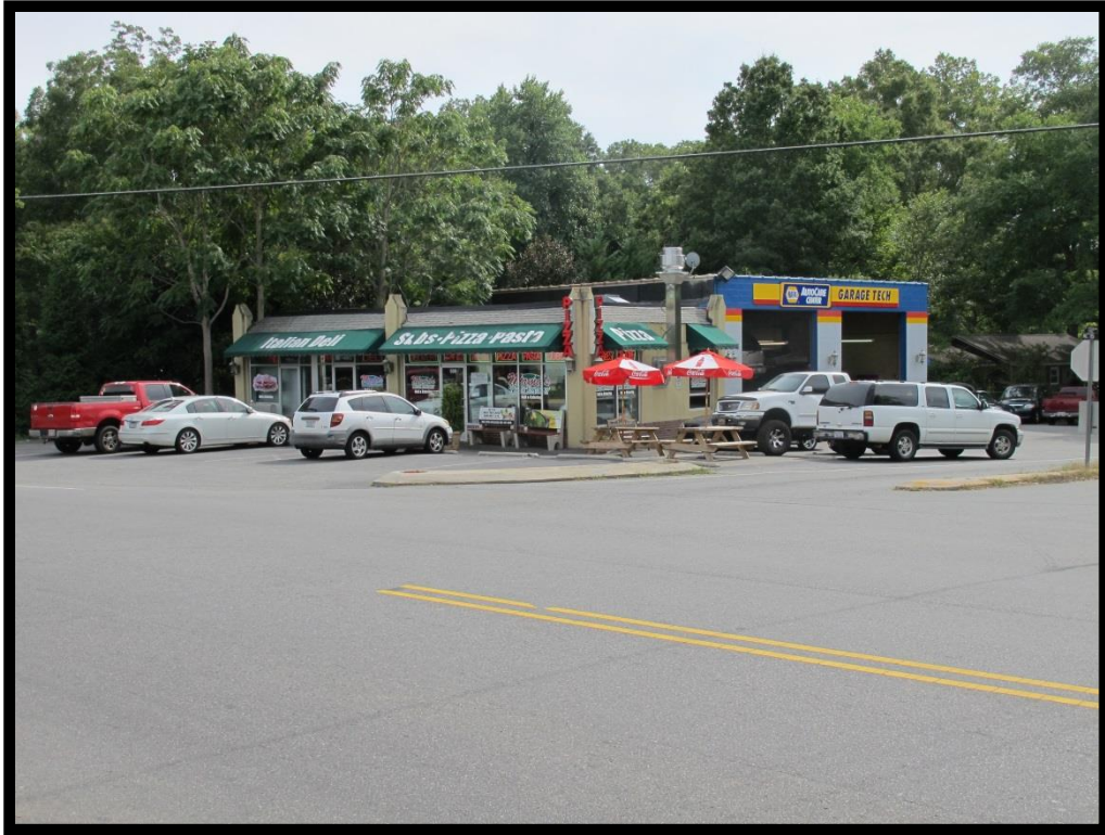
039 – View of Commercial Building/Garage, 500 S Old Statesville Rd Looking Southwest
