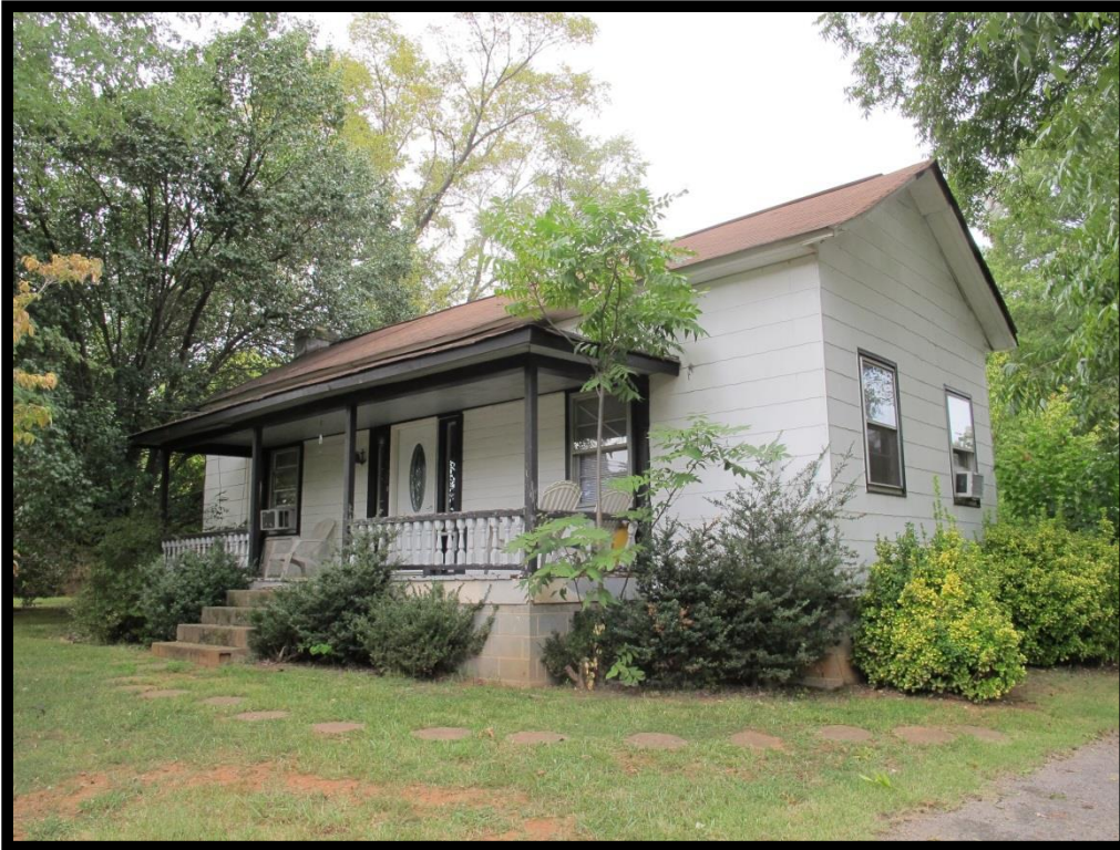
020 – View of House, 303 Huntersville-Concord Rd Looking Northwest
