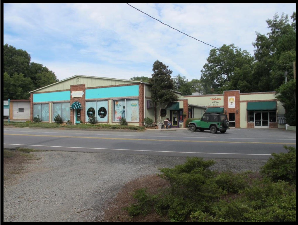
038 – View of Commercial Building, 501 S Old Statesville Rd Looking Northeast
