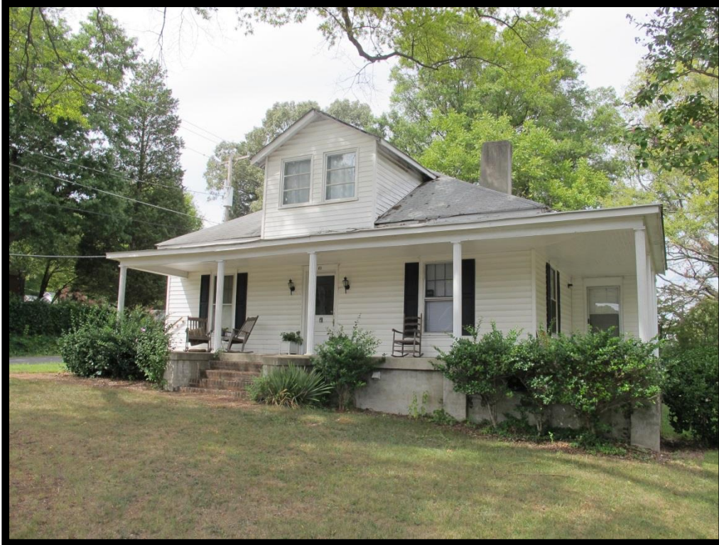
018 – View of House, 401 Huntersville-Concord Rd Looking Northwest
