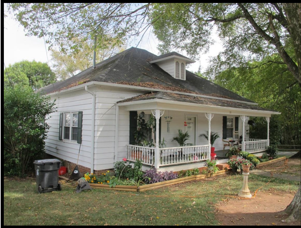
161 – View of House, 111 S. Church Street Looking Southeast
