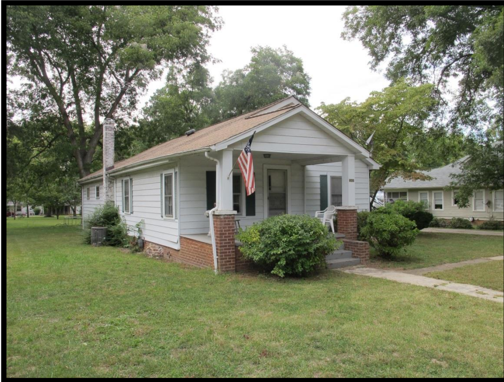
048 – View of House, 406 S Old Statesville Rd Looking Northwest
