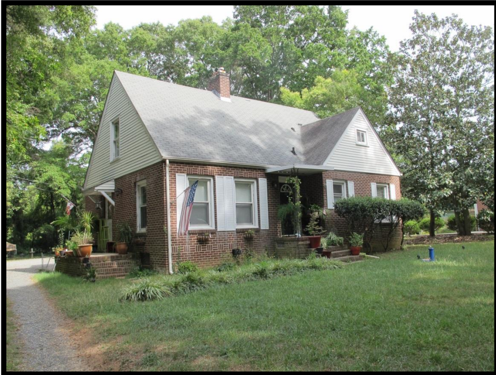
044 – View of House, 407 S Old Statesville Rd Looking Southeast
