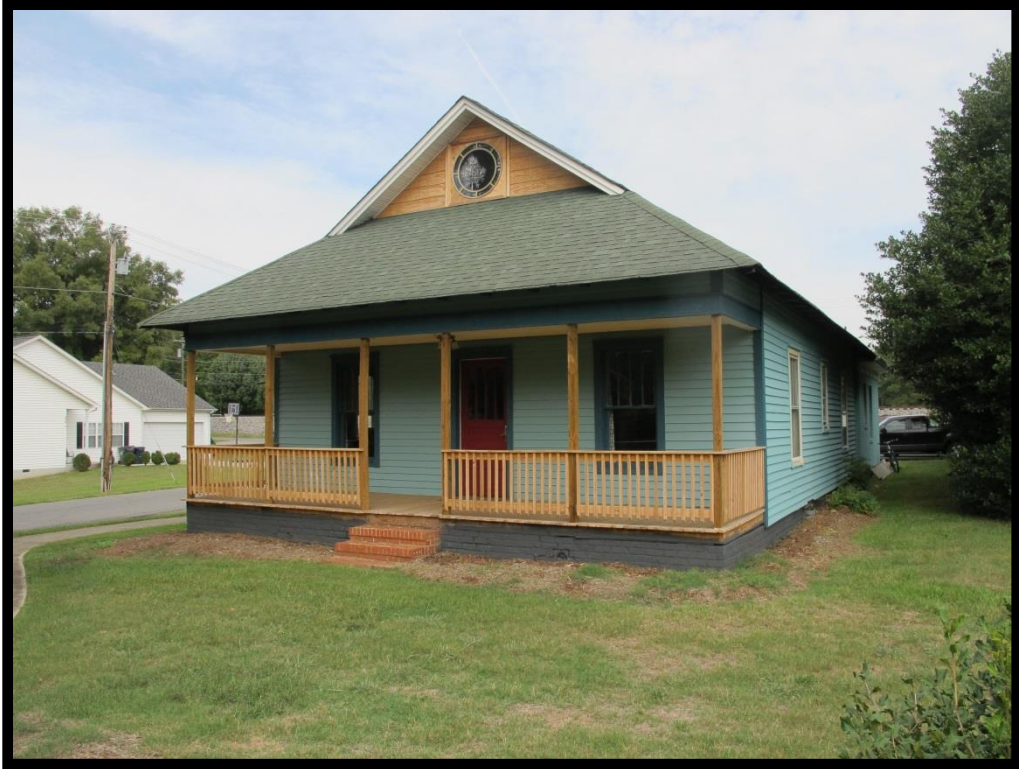
031 – View of House,13532 Old Statesville Rd Looking Northeast
