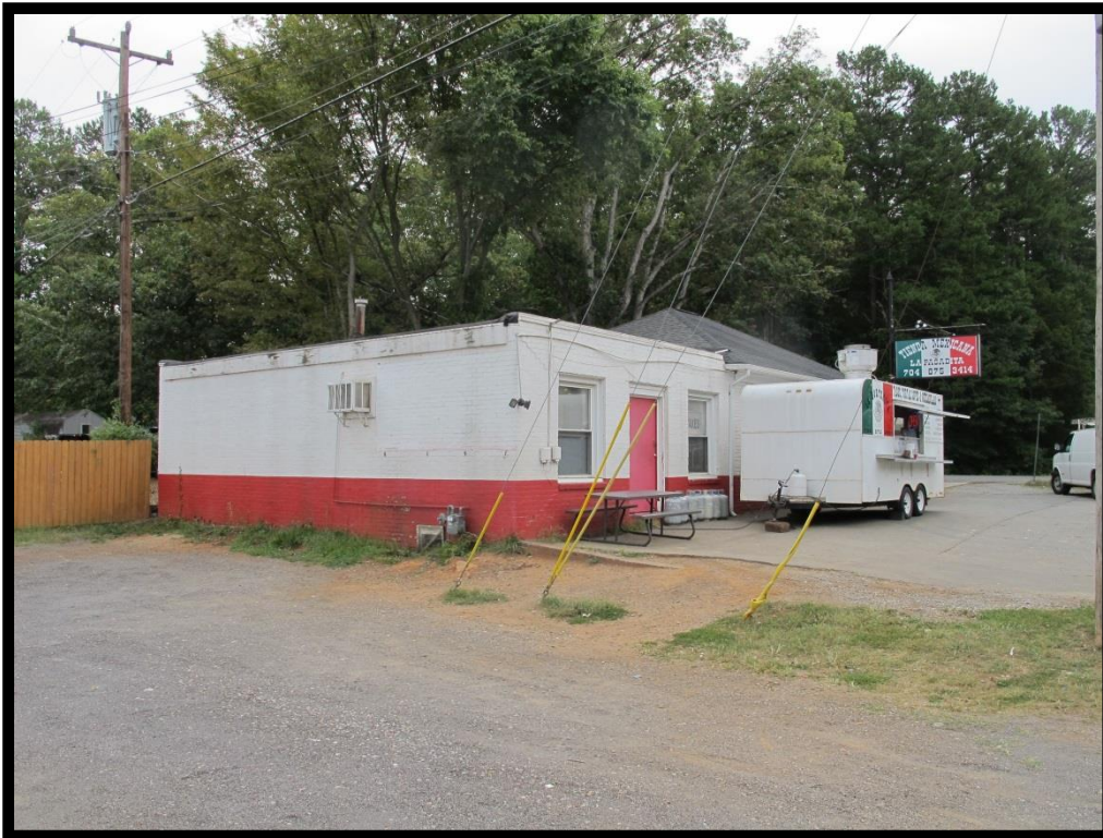
002 – View of Commercial Buildings, 500 N Old Statesville Rd Looking Southeast
