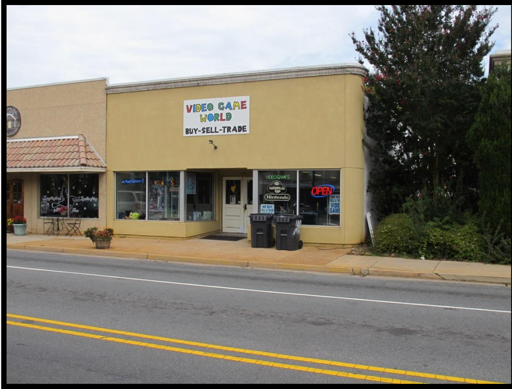
025 – View of Commercial Building, 105 S Old Statesville Rd Looking Northeast
