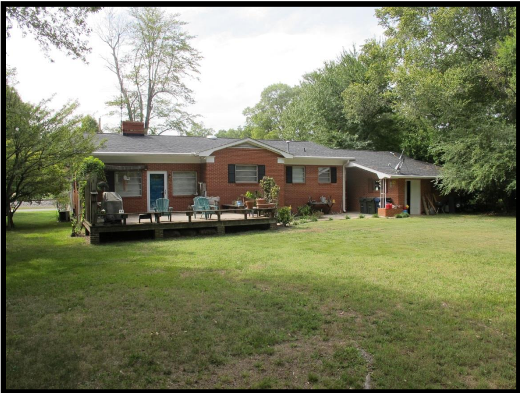
030 – View of House, 207 S Church St Looking Northwest
