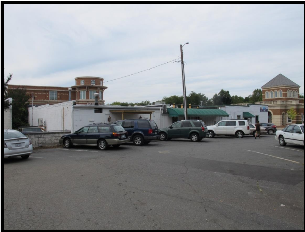
024 – View of Commercial Building, 103 S Old Statesville Rd Looking Northwest
