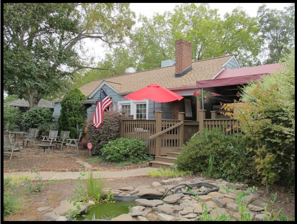
026 – View of (former) House, 100 Huntersville-Concord Rd Looking Southeast
