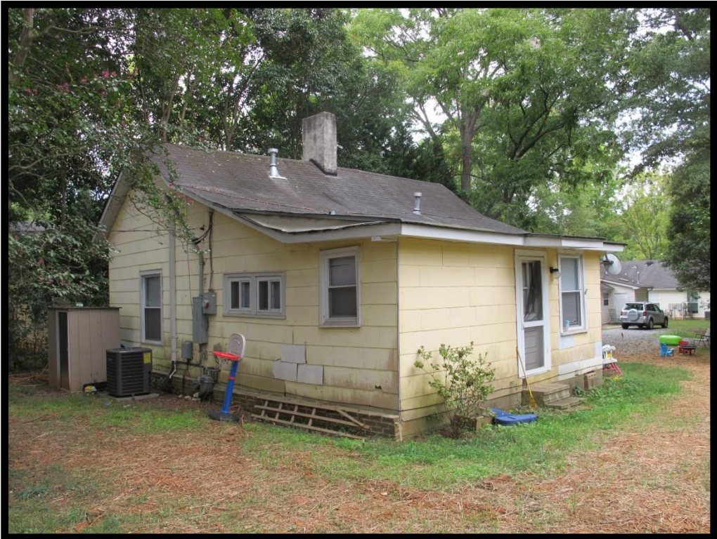
008 – View of House, 109 W Church St Looking Southwest
