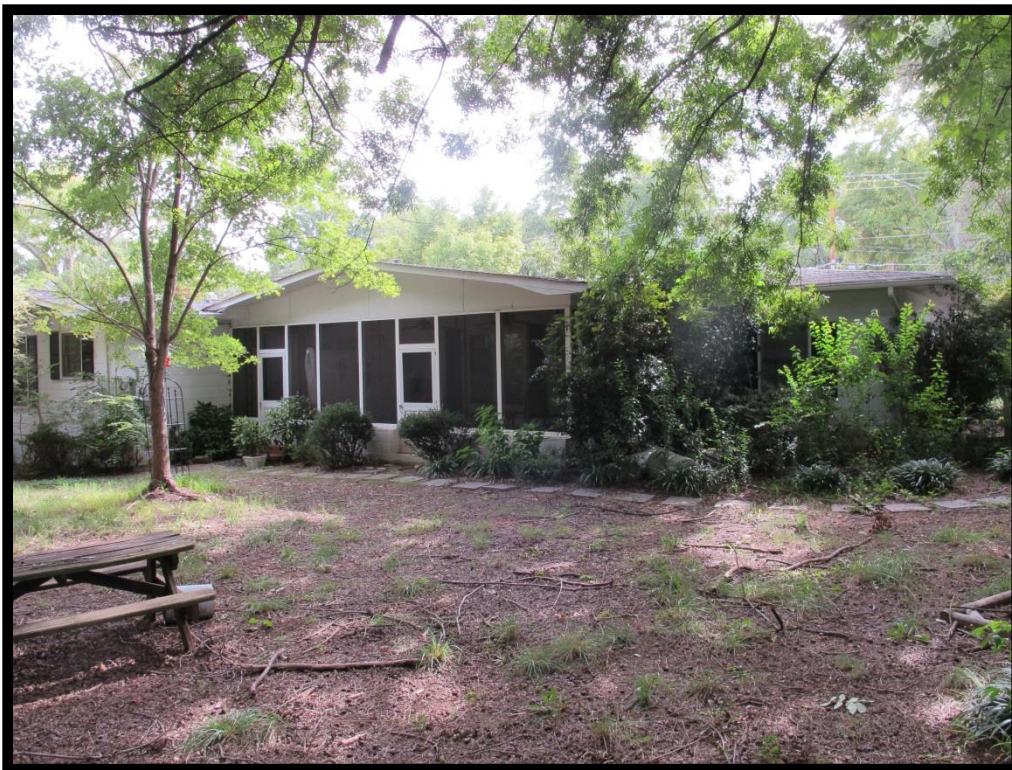
036 – View of House, 503 S Old Statesville Rd Looking South
