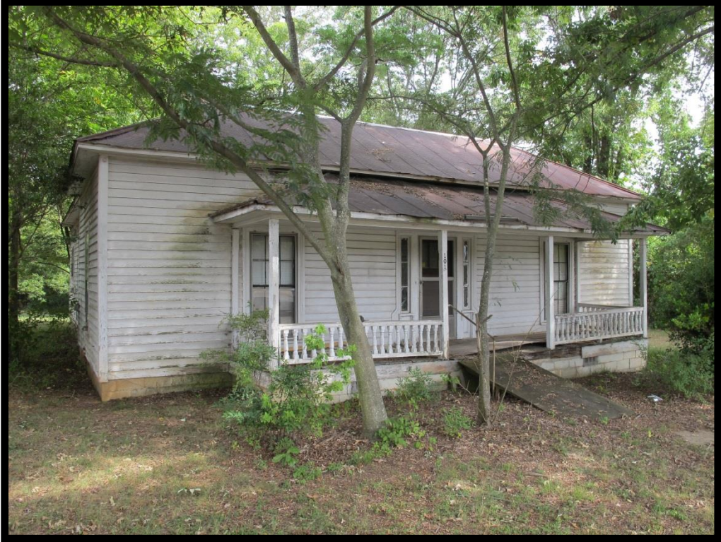
MK3084 – View of House, 101 S. Church Street Looking Southeast
