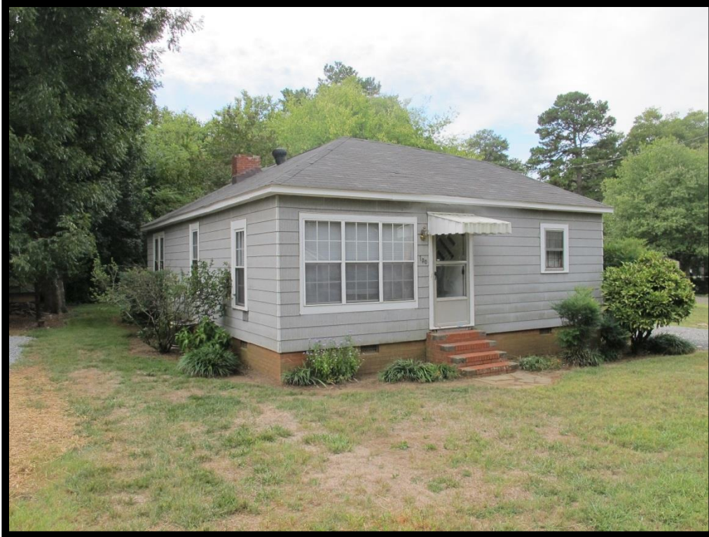
011 – View of House, 100 W Church St Looking Southwest
