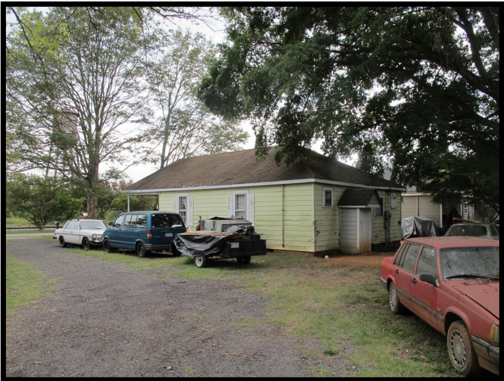
014 – View of House, 213 N Main St Looking Southeast
