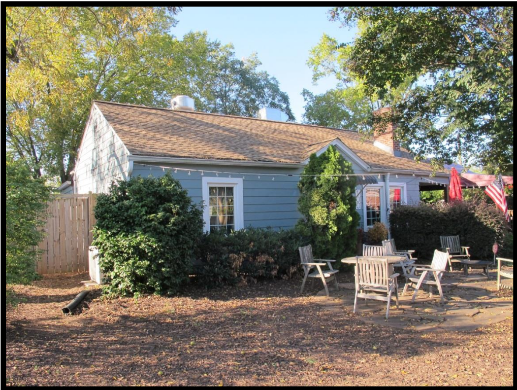
026 – View of (former) House, 100 Huntersville-Concord Rd Looking Southwest
