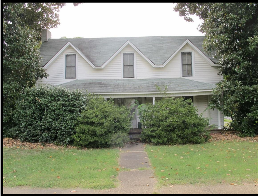
172 (MK1331) – View of Darby/McAuley House, 400 S. Main Street Looking West
