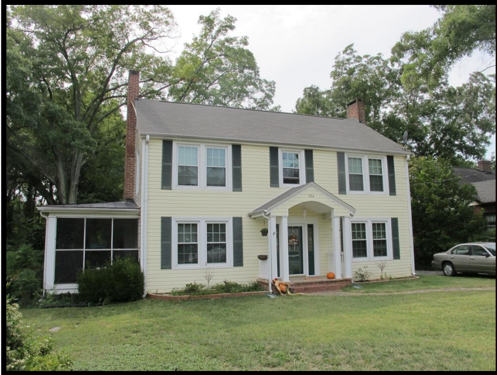
035 – View of House, 504 S Old Statesville Rd Looking West
