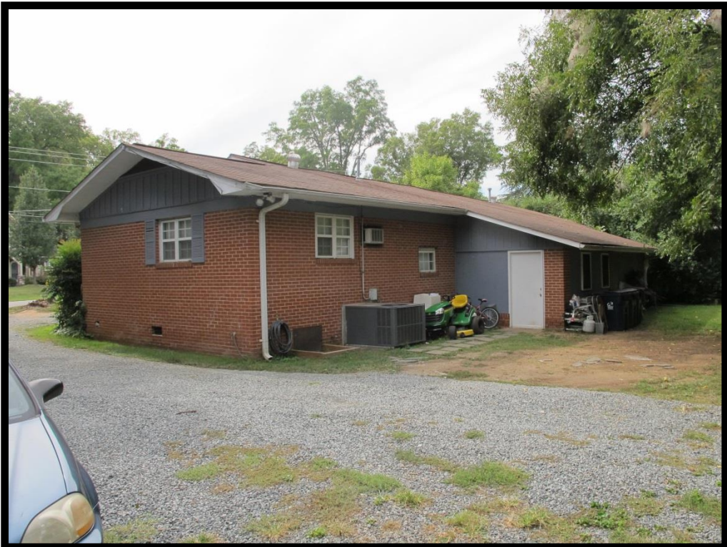
034 – View of House, 505 S Old Statesville Rd Looking Northwest
