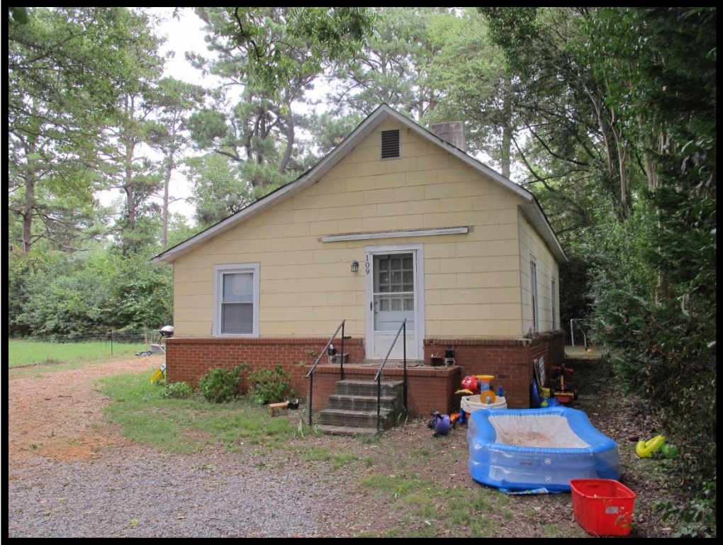
008 – View of House, 109 W Church St Looking Northeast
