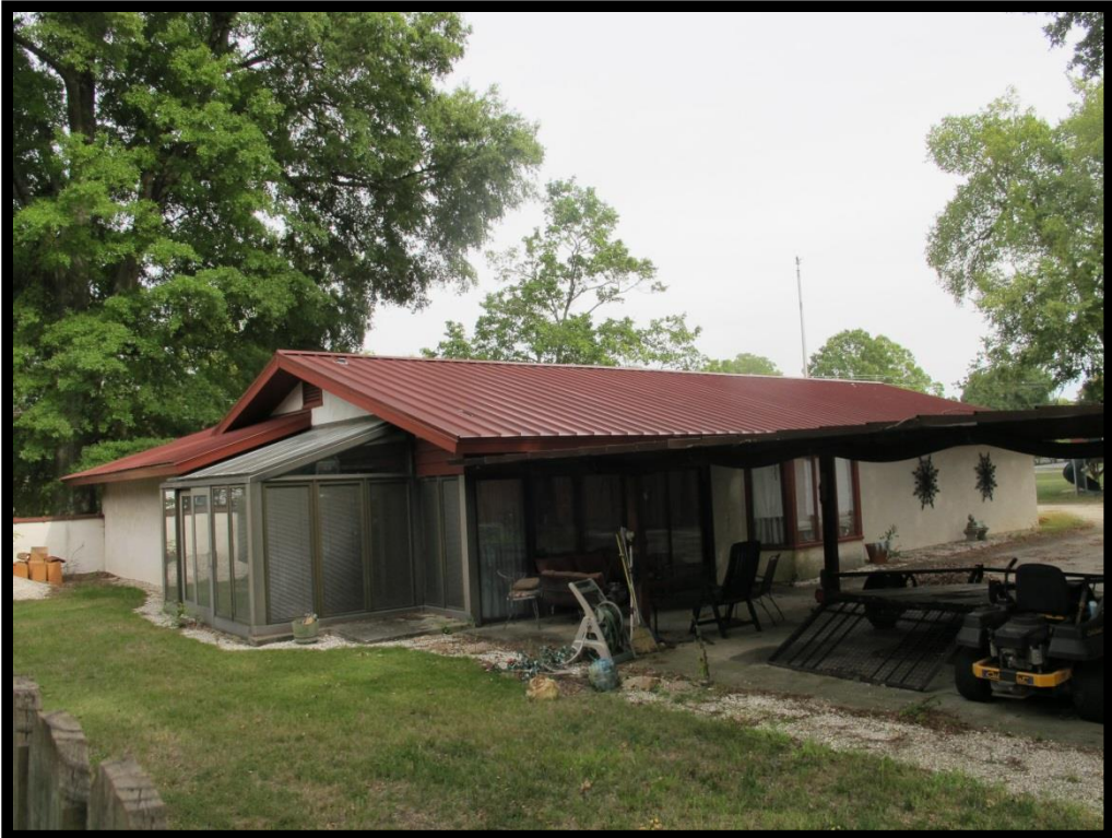
029 – View of House, 202 S Main St Looking Southeast
