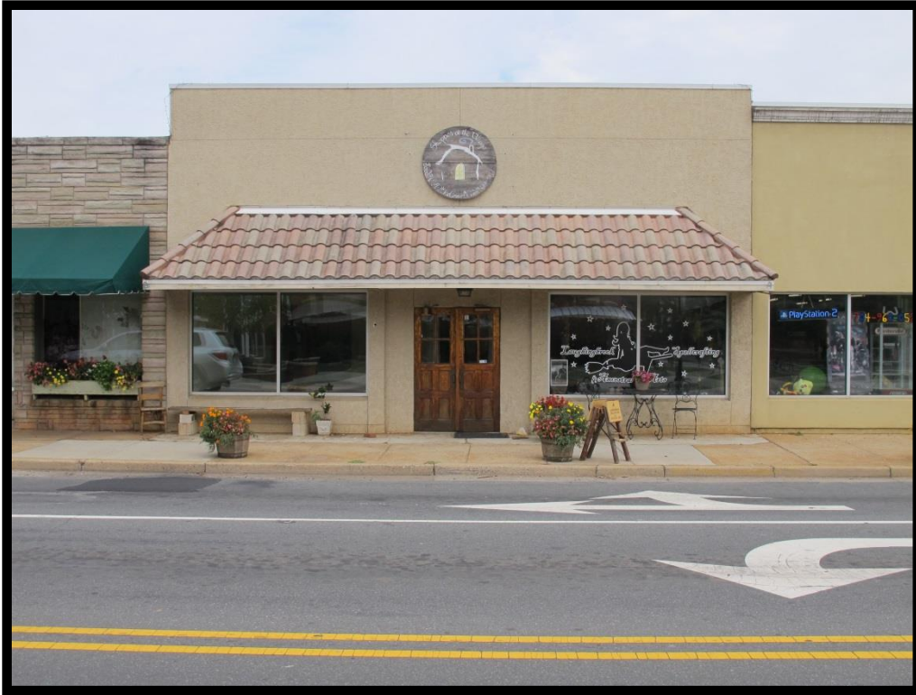
024 – View of Commercial Building, 103 S Old Statesville Rd Looking East
