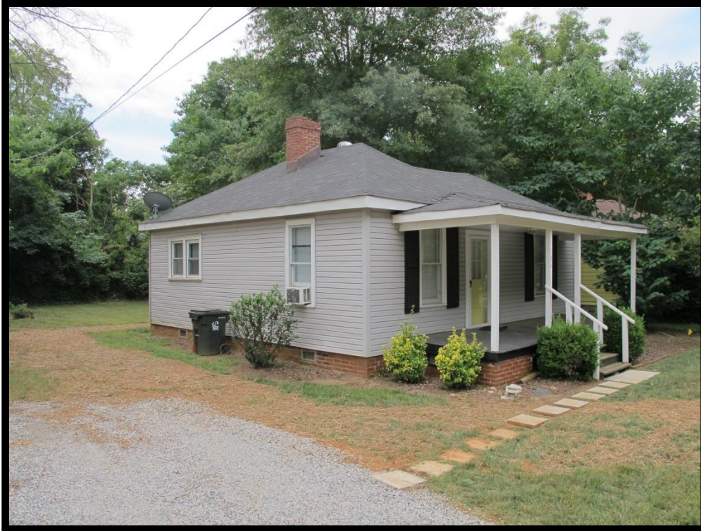
013 – View of House, 104 W Church St Looking Southwest
